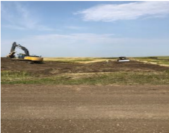
Access road being stripped - km 193+200 – Aug 2, 2018
