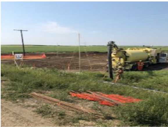
Hydrovac daylighting - Km 183+989 – Aug 3, 2018
