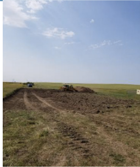
Moving topsoil – km 193+000, Aug 1, 2018
