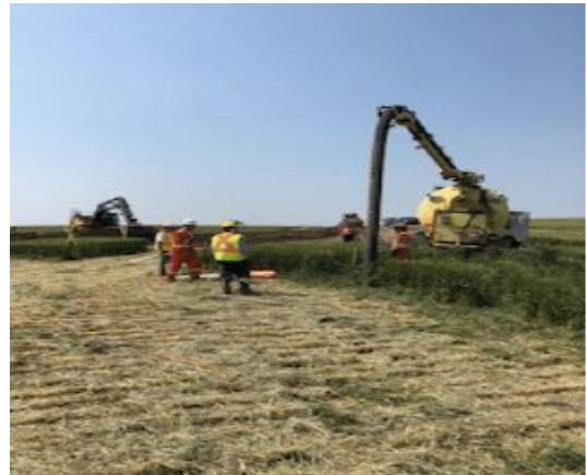
Hotline being daylighted - km 192+800 – Aug 2, 2018
