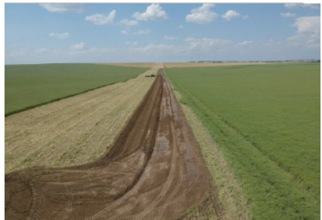
Grader and tractor stripping topsoil - Km 173+000 – Aug 3, 2018
